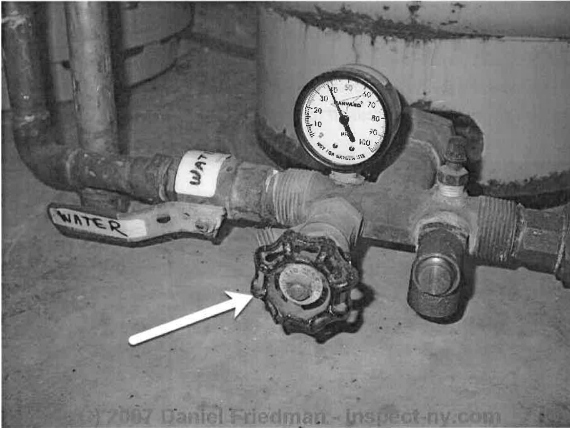
A main water shutoff valve, in this case the blue lever labeled "WATER" with white tape, is shown to the left of the pressure gauge and pressure tank drain valve in our photograph (white arrow).
