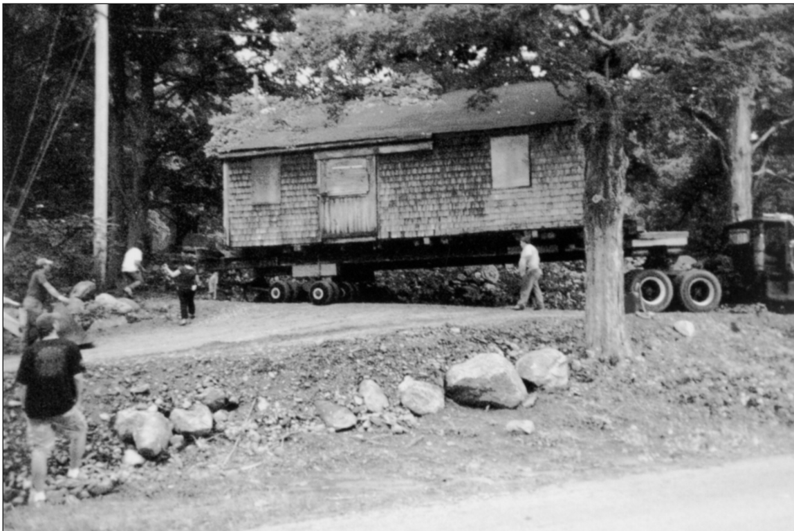
POSITIONING THE BUILDING AT THE NEW SITE
