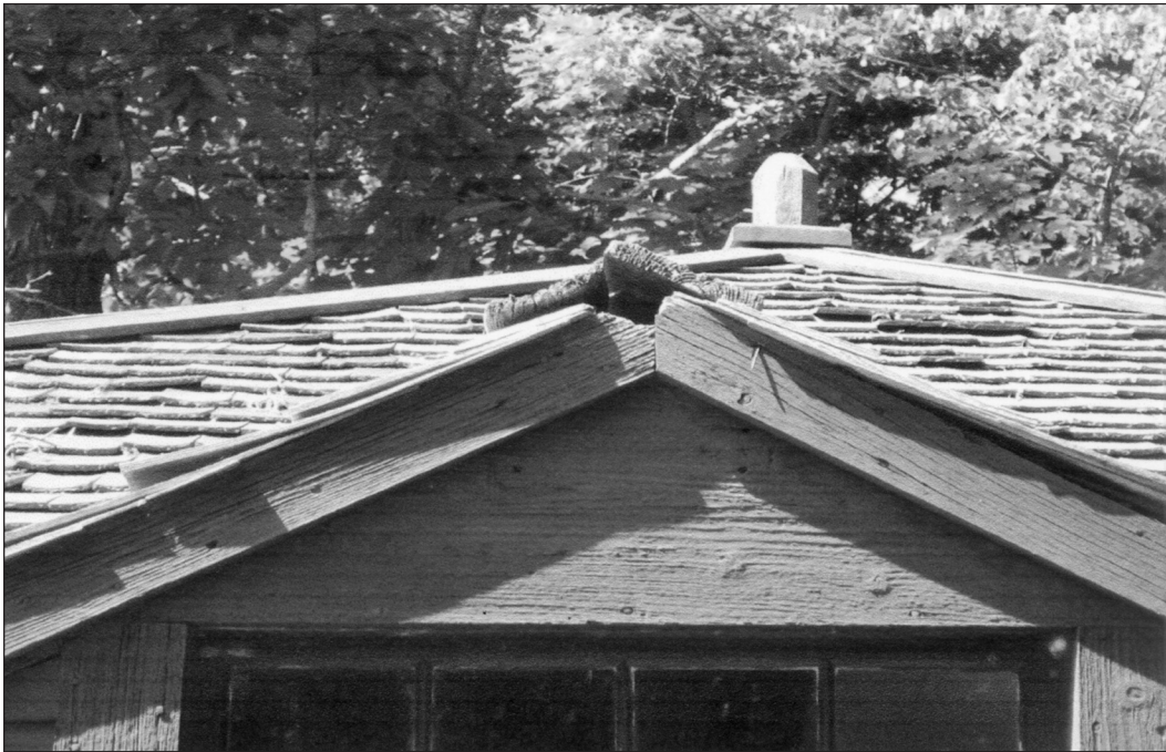
Squirrel hole on entryway's facier board at peak
